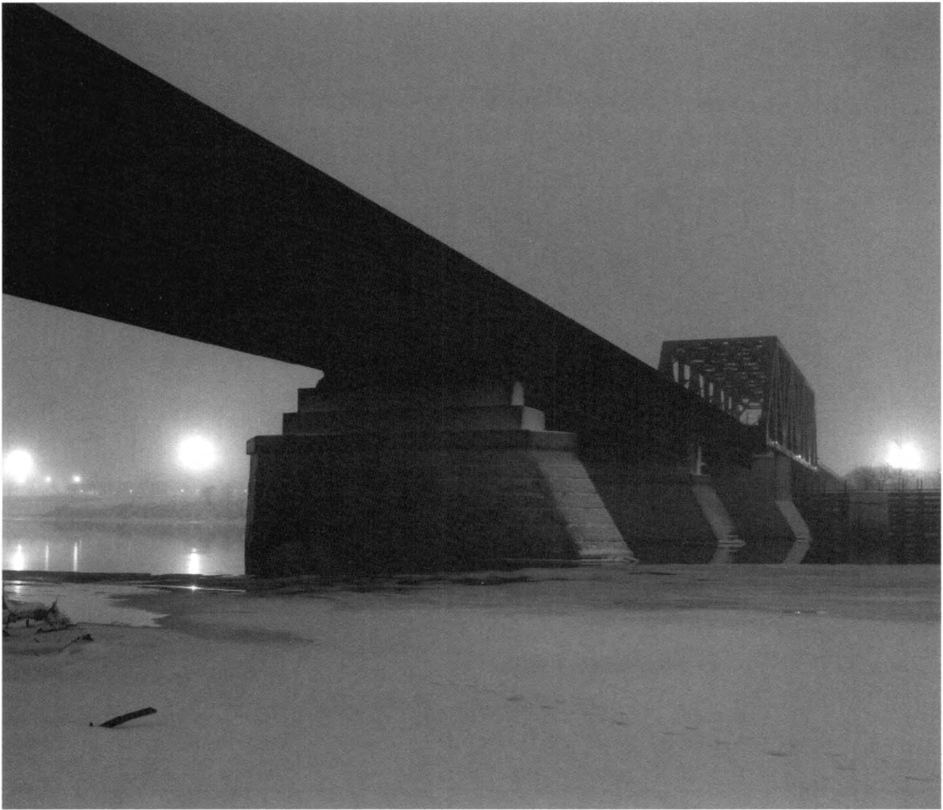
SOO LINE RAILROAD BRIDGE ACROSS THE MISSISSIPPI RIVER, NORTHEAST MINNEAPOLIS, 1996
